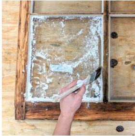
49. Gently using a brush against the putty to pick up oily residue
