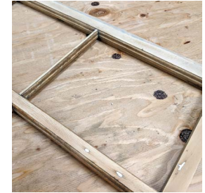
20. Holes filled with Abatron WoodEpoxy
