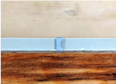
35. A point not pushed into the sash far enough
