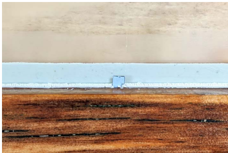
36. A point properly pushed into the sash
