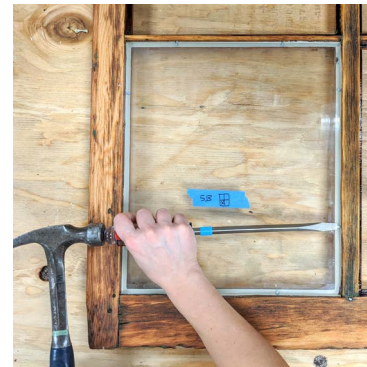
38. Tapping glazing points into sash with a screwdriver and hammer
