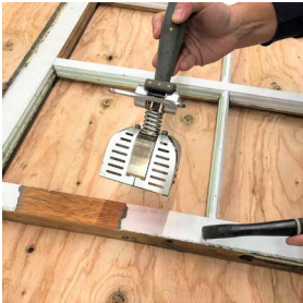
12. Heating paint to be scraped
