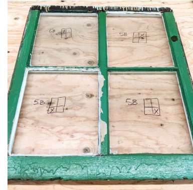
8. Panes of glass labeled with window number and location of glass within the sash
