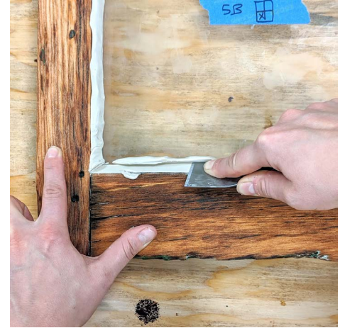
41. Spreading the putty into a clean, smooth line
