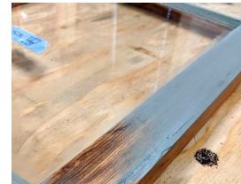
46. Painting a THIN coat of linseed oil paint
