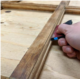
17. Sanding the profiles with a contour grip
