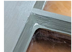
47. Too much paint in the corner that will not dry properly
