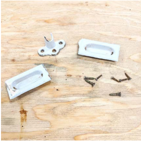
10. Handles and locking mechanism removed from sash
