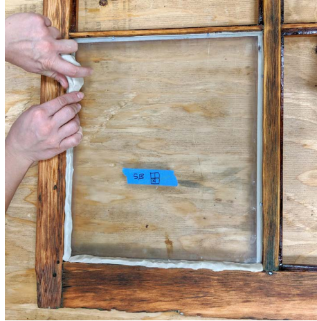
40. Pressing glazing putty in around the perimeter
