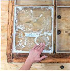
48. Using fingers to rub whiting over the glass to pick up leftover oily residue
