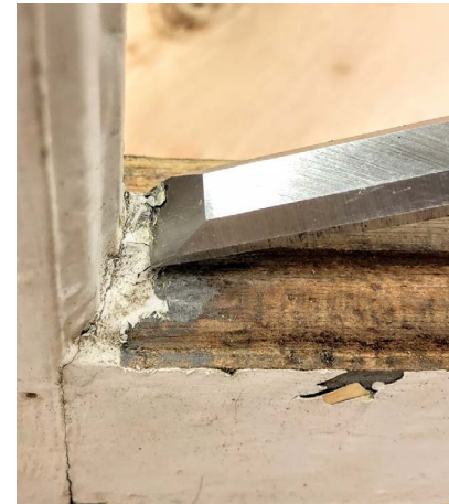
14. Using a curved scraper for the profiles
