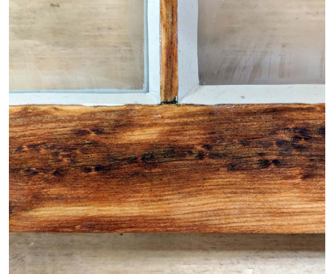
43. Glazing properly inside the edge on the left, while the right side needs to be pulled in a bit more
