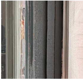
51. Failing glazing putty that should be repaired
