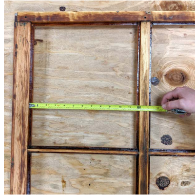
26. Measuring for a new pane of glass
