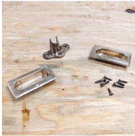
11. Many layers of paint removed from hardware via boiling water and baking soda
