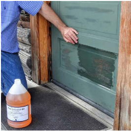
50. Wiping raw linseed oil over linseed oil paint that needs to be rehydrated [photo courtesy of the National Park Service]
