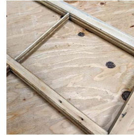
19. Small holes to be filled with epoxy
