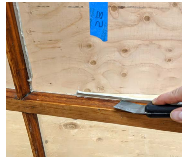
39. Cleaning off the oozing glazing on the underside of the glass
