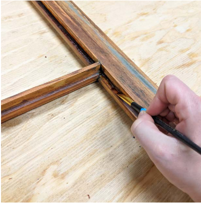
24. Using a small paintbrush to apply shellac to glazing beds
