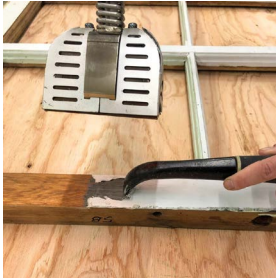
13. Paint being scraped with infrared heater
