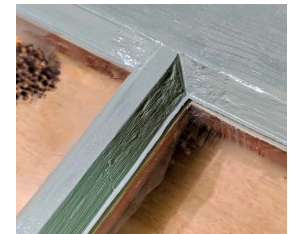
45. Paint properly applied 1/16" onto the glass
