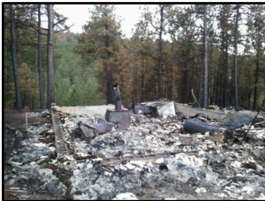
Figure 11. A site where mitigation had not been done, resulting in a total loss of the structure. Note that several trees in the immediate vicinity have not been burned, suggesting the likelihood that embers may have been the ignition source.
