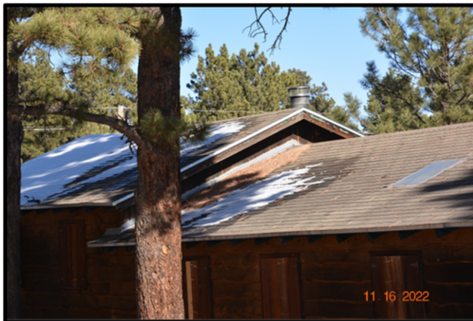
Figure 5. Pine needles that have accumulated on the roof below the soffit and fascia that are susceptible to ignition from embers. The flames could easily spread to the wood soffit and fascia.
