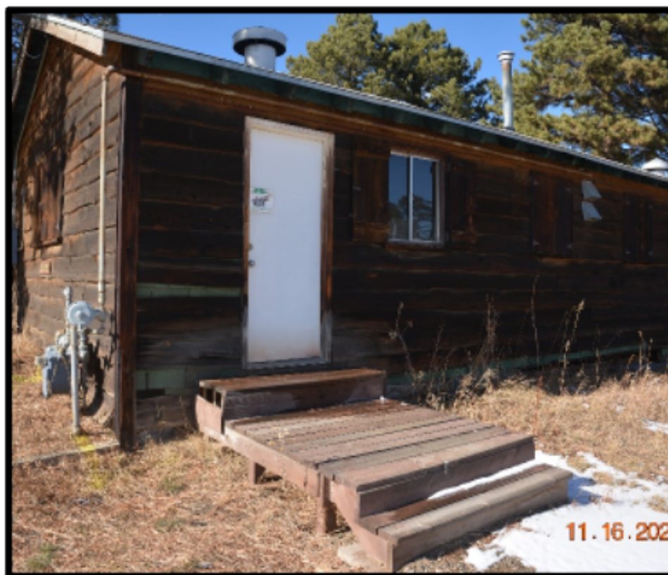
Figure 6. Wooden stairs in contact with ground vegetation provide a source for spread of the fire from surface fuels to the wood structure.
