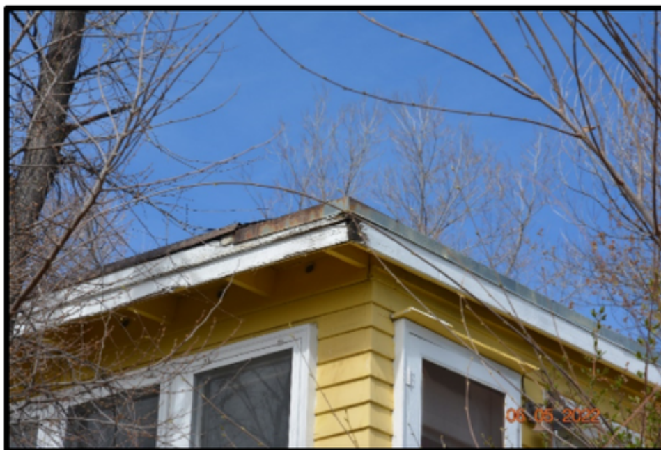
Figure 7. Deteriorated fascia board that provides an entry for wind-driven embers can result in an ignition on the interior of the structure.
