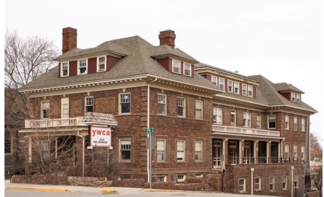
Figure 1 The Helena YWCA building was rehabilitated in 2016 with $118,000 in MHTCs and $470,000 in HTCs. It meets a critical social need with transitional housing and supportive services for homeless women and their children. Photo credit: Diamond Construction.
