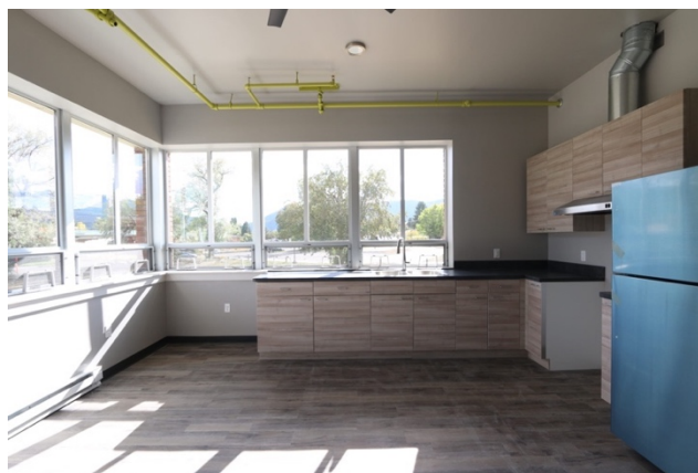
Figure 11 Interior renovation of hospital space to residential space at the Livingston Memorial Hospital. Photo credit: Homeword.
